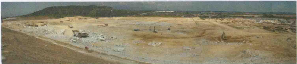
EARTHWORKS & BLASTING SPECIALIST CONSTRUCTION
